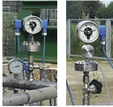
Before (left): mechanical pressure transmitter with bourdon tube. After (right): digital pressure transmitter with mechanical gauge.
